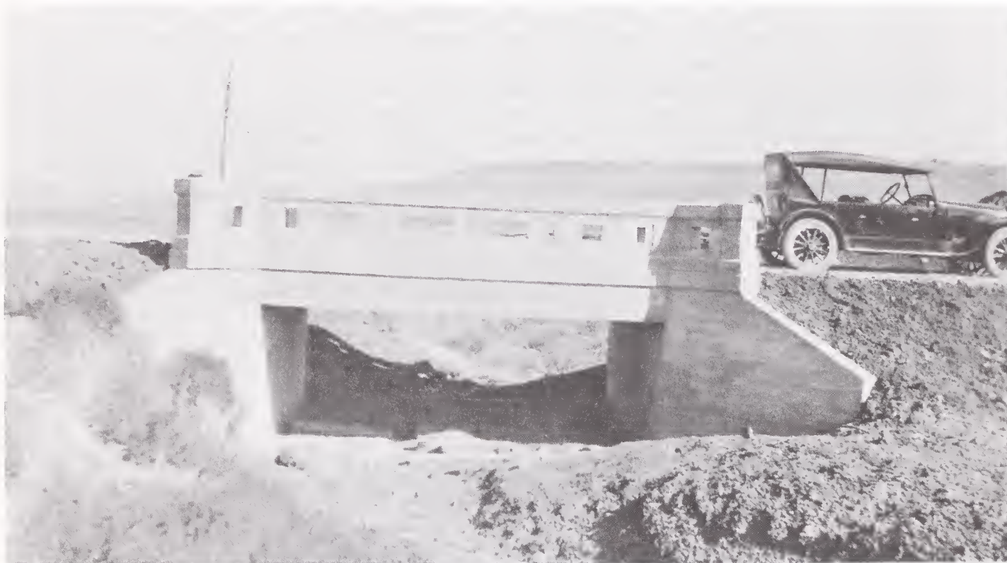
Montana Highway Commission reinforced concrete slab bridge, circa 1930.
